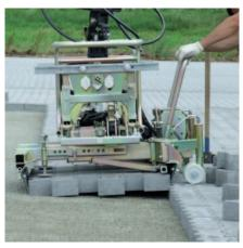
Slab grab used in combination with excavator
