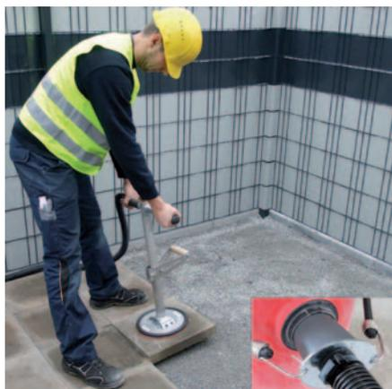
Efficient and accurate installation of small-sized and lightweight slabs – this is the optimum application enhancement for the vacuum devices QUICKJET QJ-600-E and SPEEDY VS-140/200.
